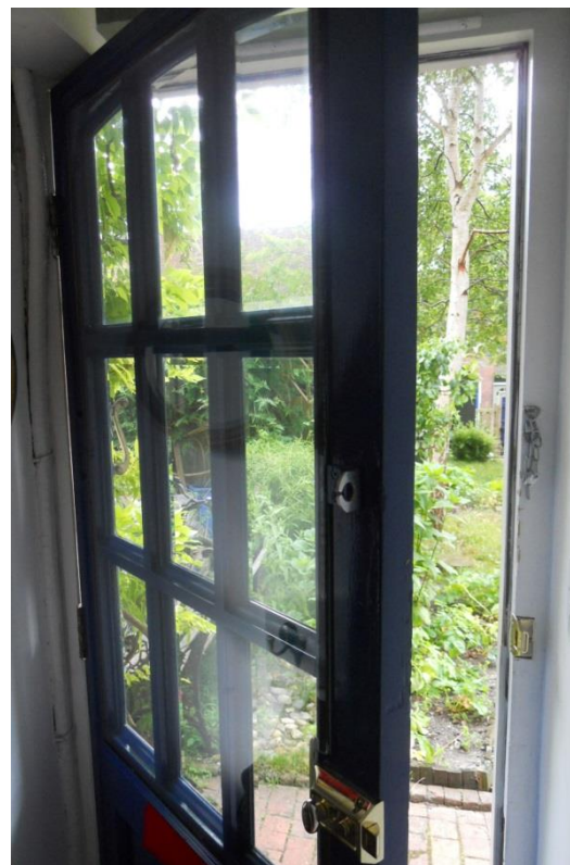
Magnetic-strip glass secondary glazing on front door ↓
