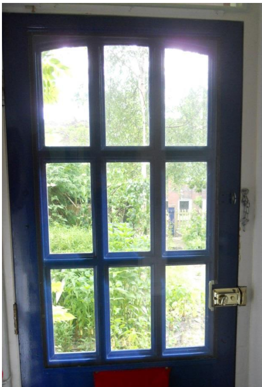
Magnetic-strip glass secondary glazing on front door ↓
