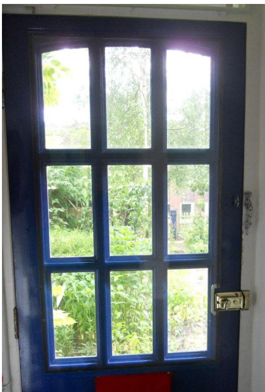
Magnetic-strip glass secondary glazing on front door ↓
