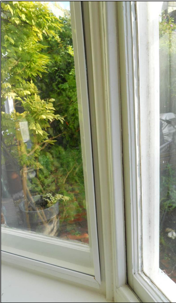
Magnetic-strip glass secondary glazing on non-opening sash window ↑
