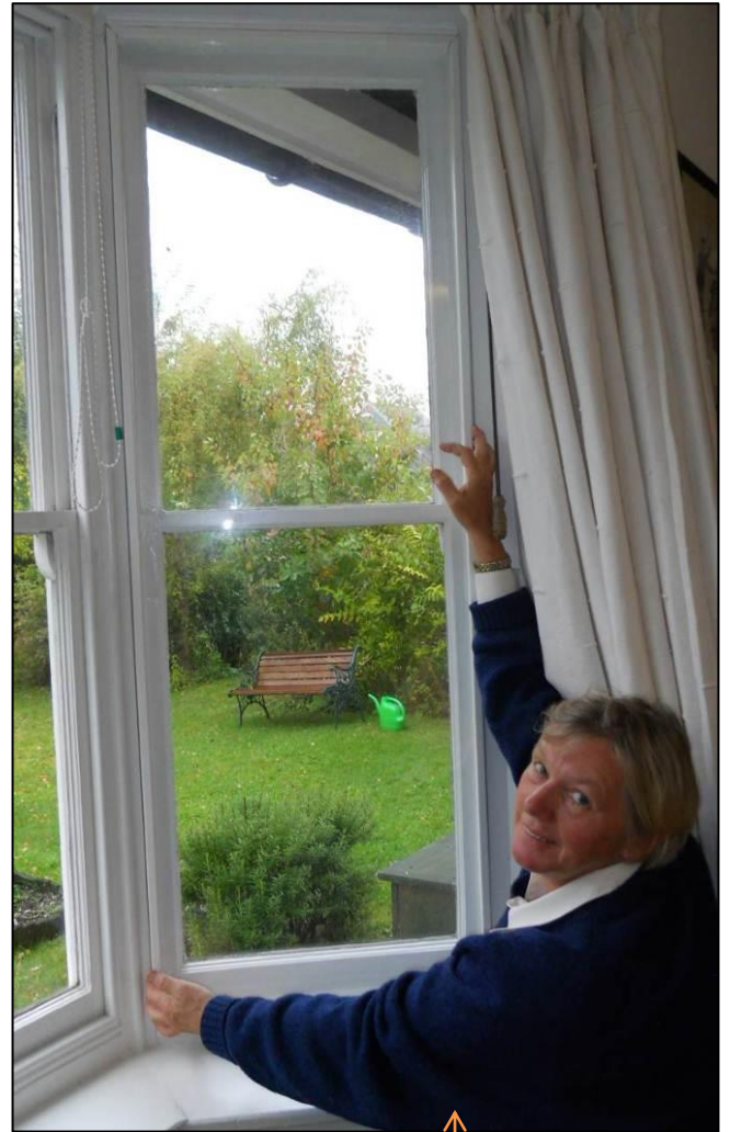
Magnetic-strip glass secondary glazing on non-opening sash window ↑
