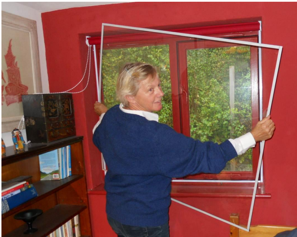
Magnetic-strip acrylic secondary glazing on modern wooden windows
