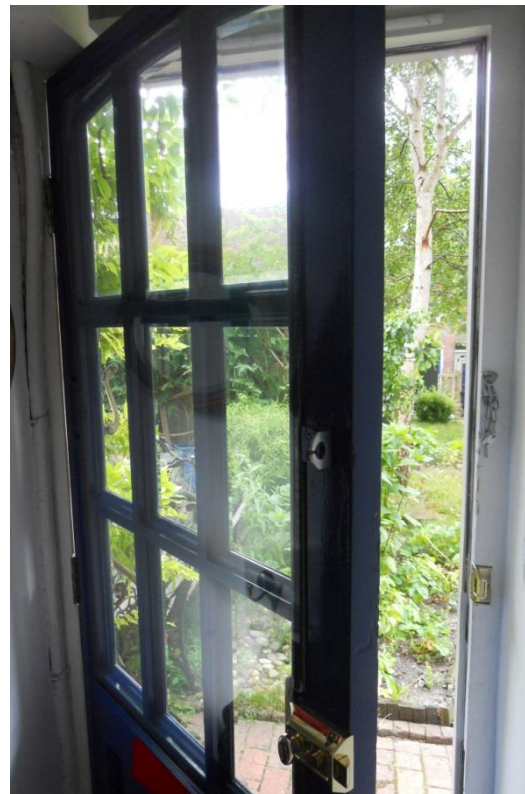
Magnetic-strip glass secondary glazing on front door ↓
