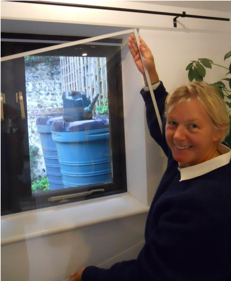
Magnetic-strip acrylic secondary glazing on modern wooden windows
