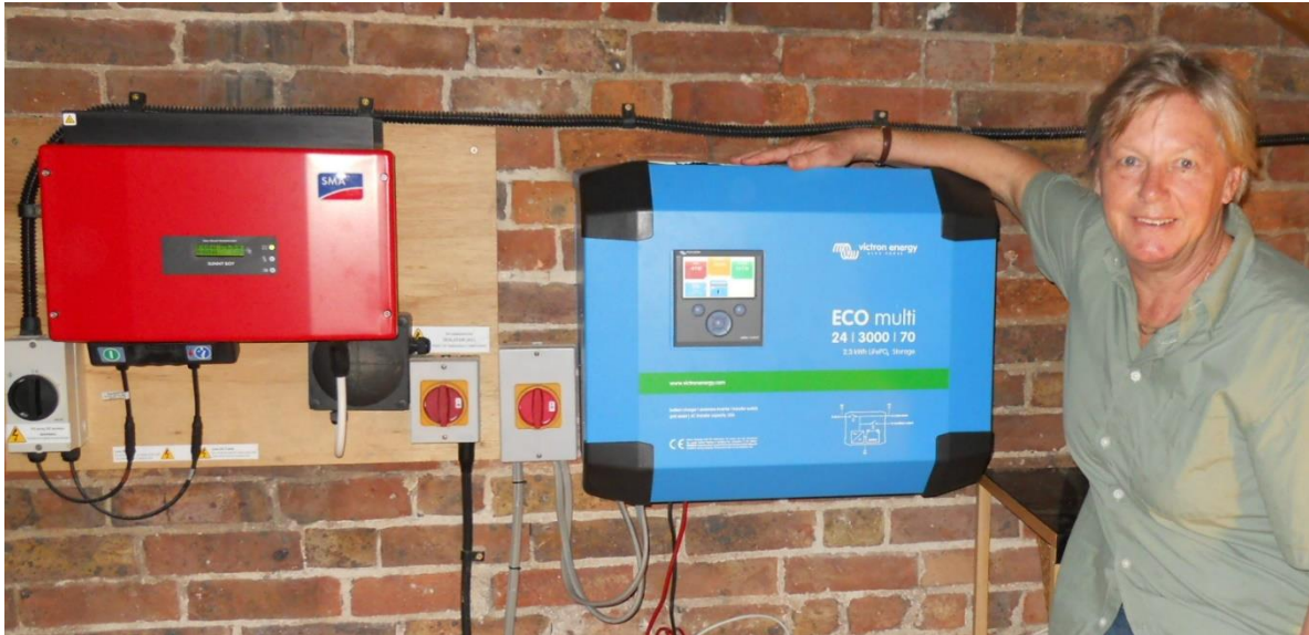
Jill with her solar panel and lithium storage battery installations
