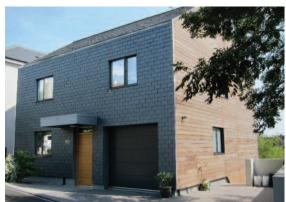
The roof is particularly interesting with integrated Solar Thermal and PV panels, coupled with opening skylights which fill the upper rooms with light. These renewables have Bluetooth output to give fascinatingly detailed data on performance. The external appearance is handsomely finished in slate at the front, with timber cladding wrapping round the sides and back
